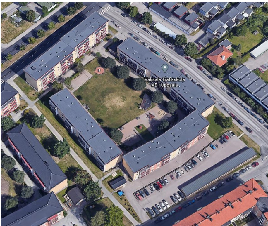
Figur 18: Fastigheten via Google earth
