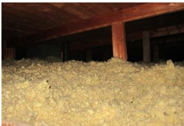
Figur 23: Takisolering 400-500mm tjock
